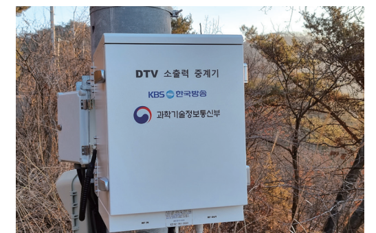
▲ Resolving irregular reception with low-power repeater
